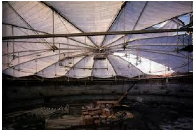
Fig. 2.1. Olympic Hall roof in Seoul during the construction [132]
